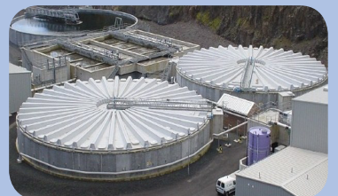
↑ Bonding GRP sewage covers
